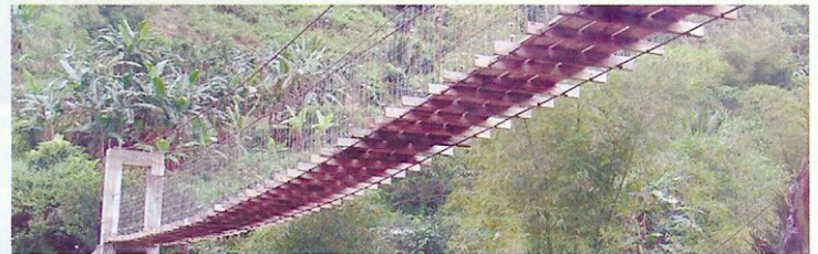
A swinging bridge traversing a stream at Runruno.
