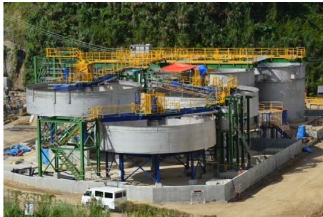
Image 9: CCD Thickener area
