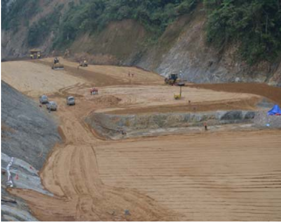
Image 11: RSI clay core construction of the dam wall
