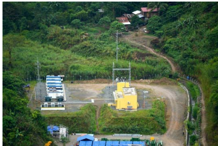
Image 2: Switchyard aerial view
