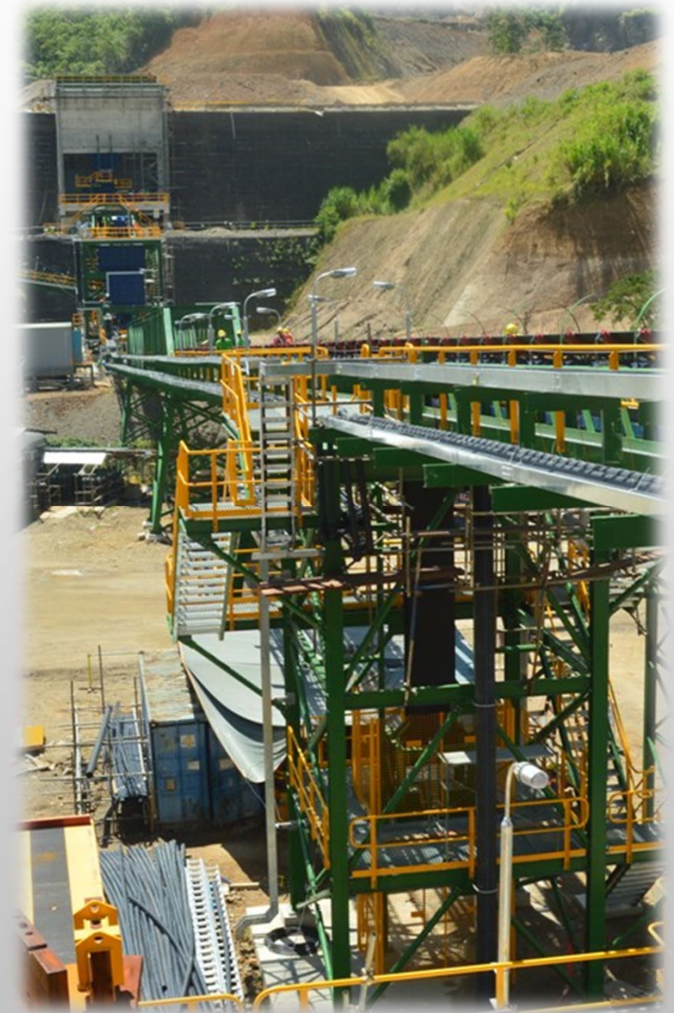
Crusher, transfer station and ore conveyor
