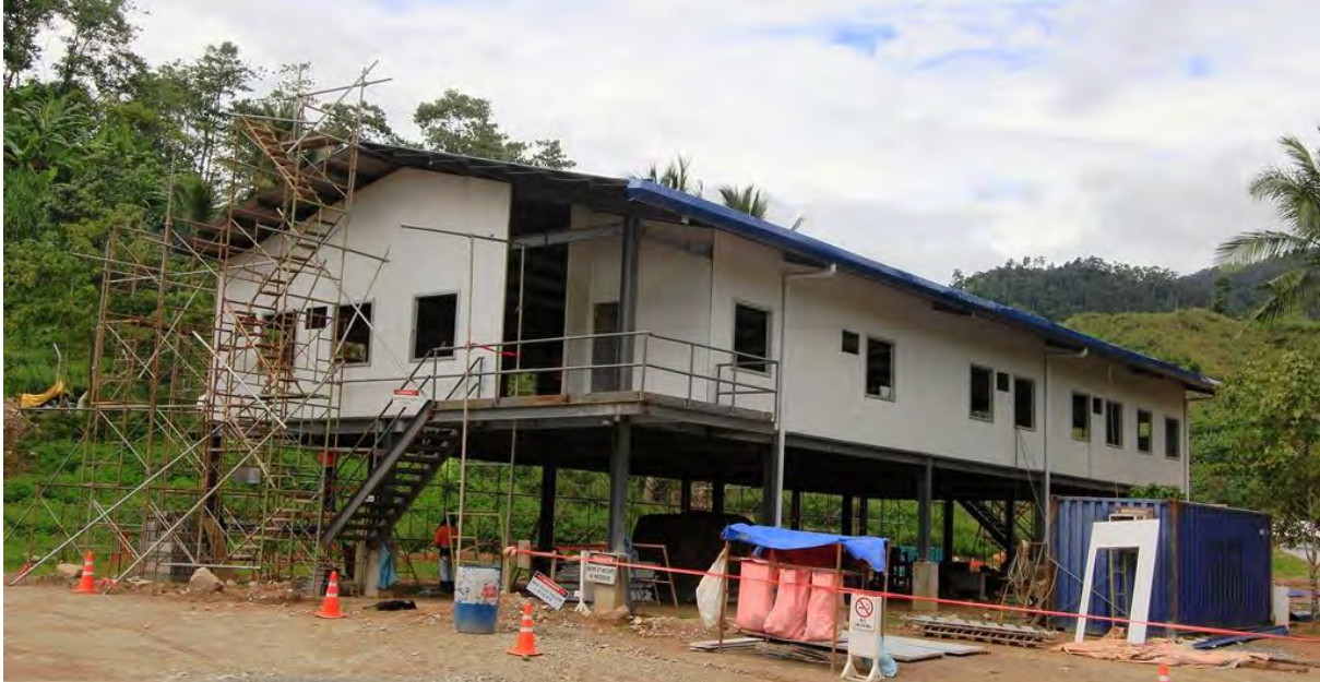
Two storey office block - in construction
