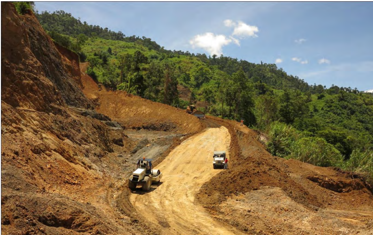
Development of pit access road - looking towards starter pit location
