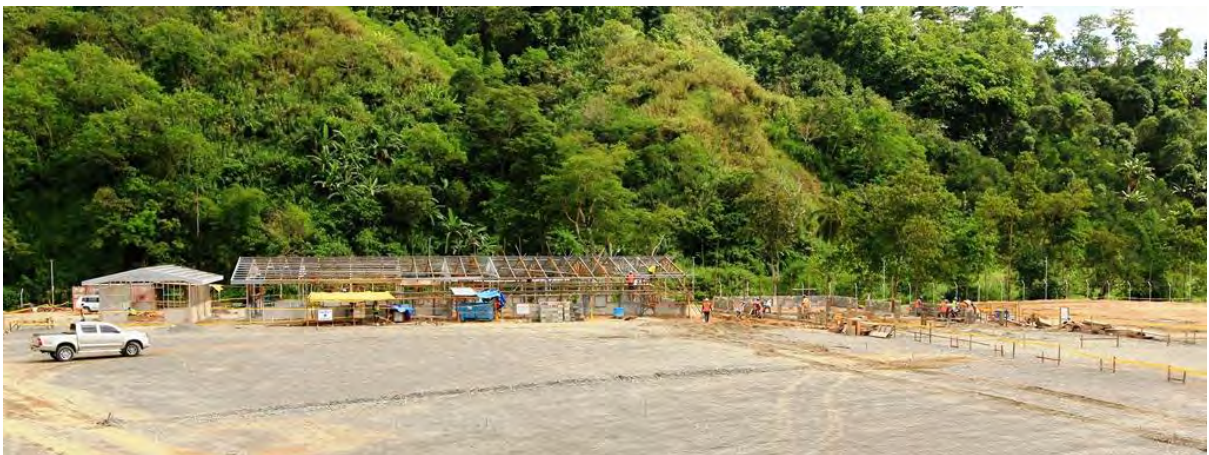
Stage 1 of construction camp - ablutions, accommodation and messing facilities
