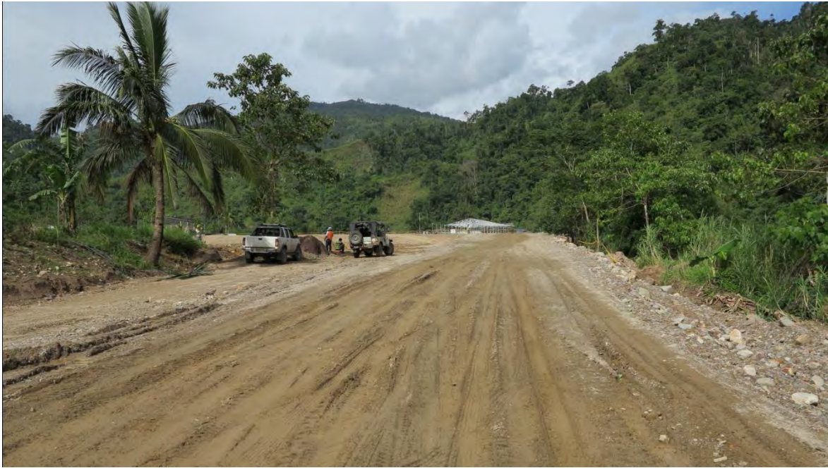
Site access road - looking towards campsite and lay-down area
