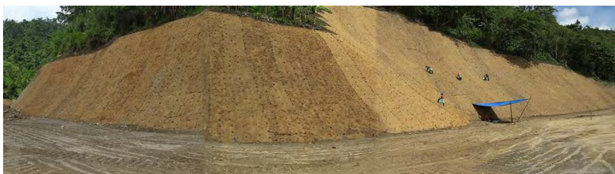
Rehabilitation of cut slopes in the processing plant area using coconut matting and napier grass
