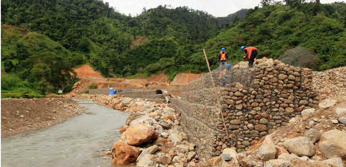
Gabion wall construction - processing plant
