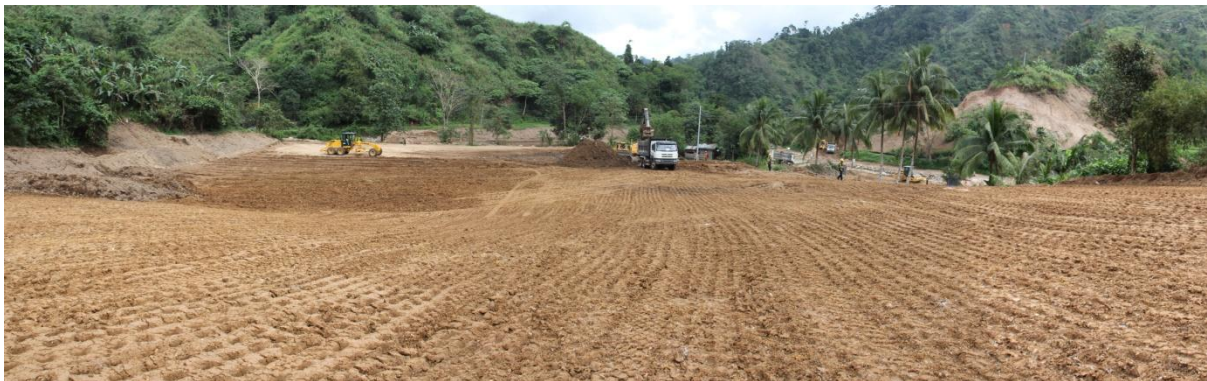
Processing plant site earthworks - looking north (20 Jan 2012)
