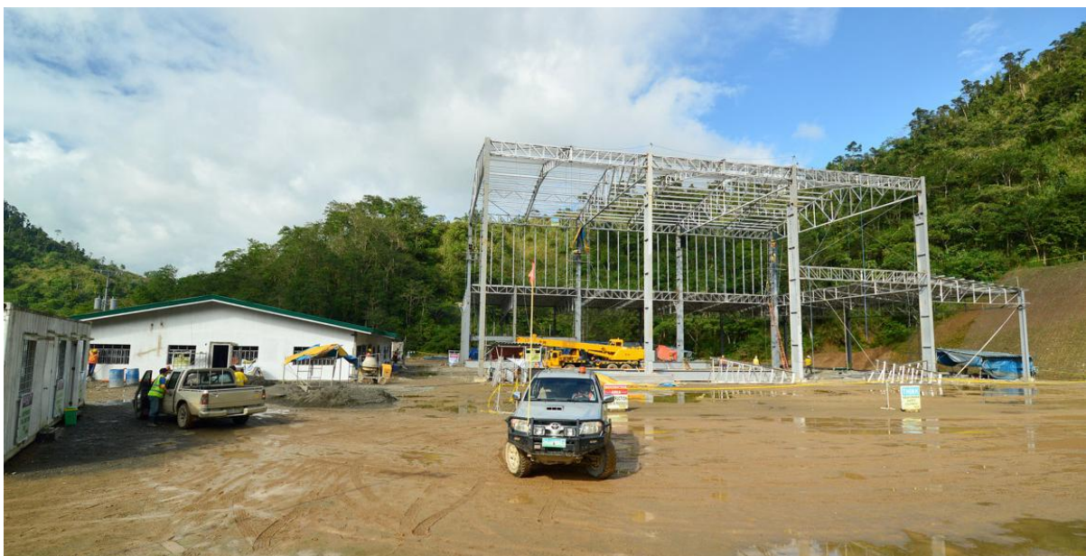
Image 7. Heavy vehicle workshop and mine office construction activities
