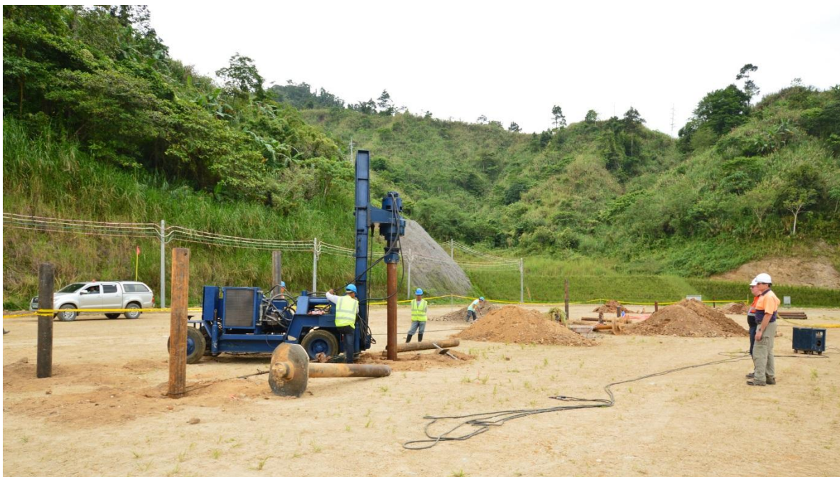
Image 13: Screw piling works
