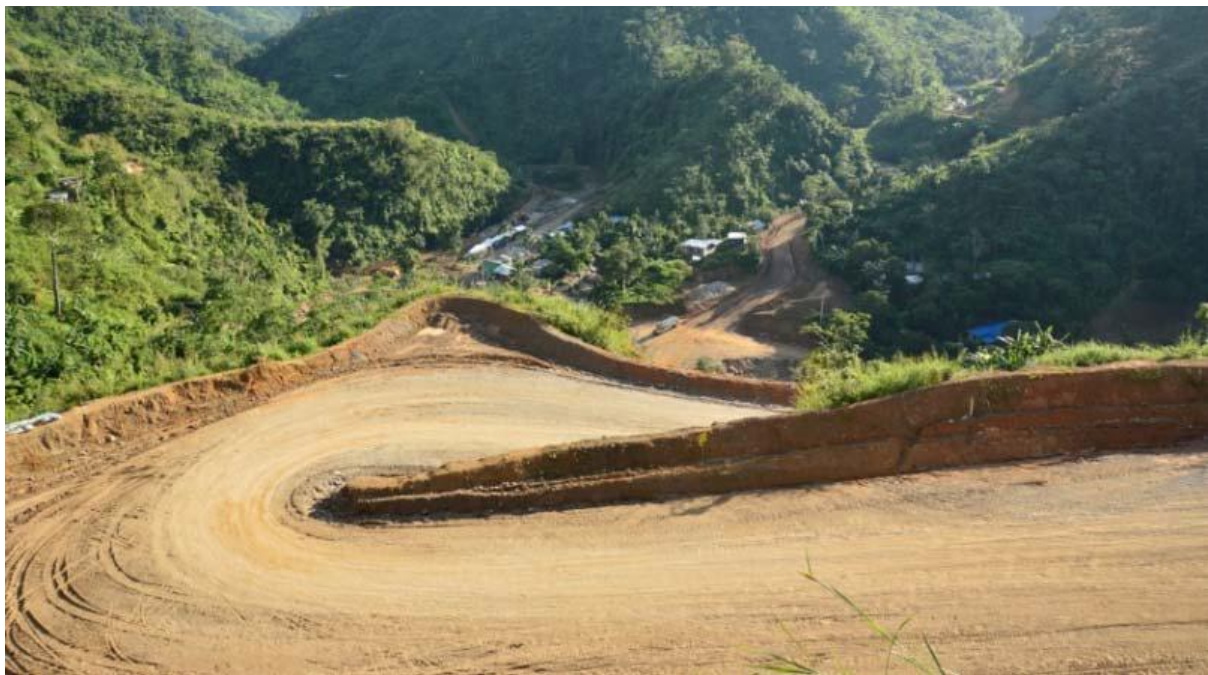
Image 9: Mine haul road into Residual Storage Impoundment site
