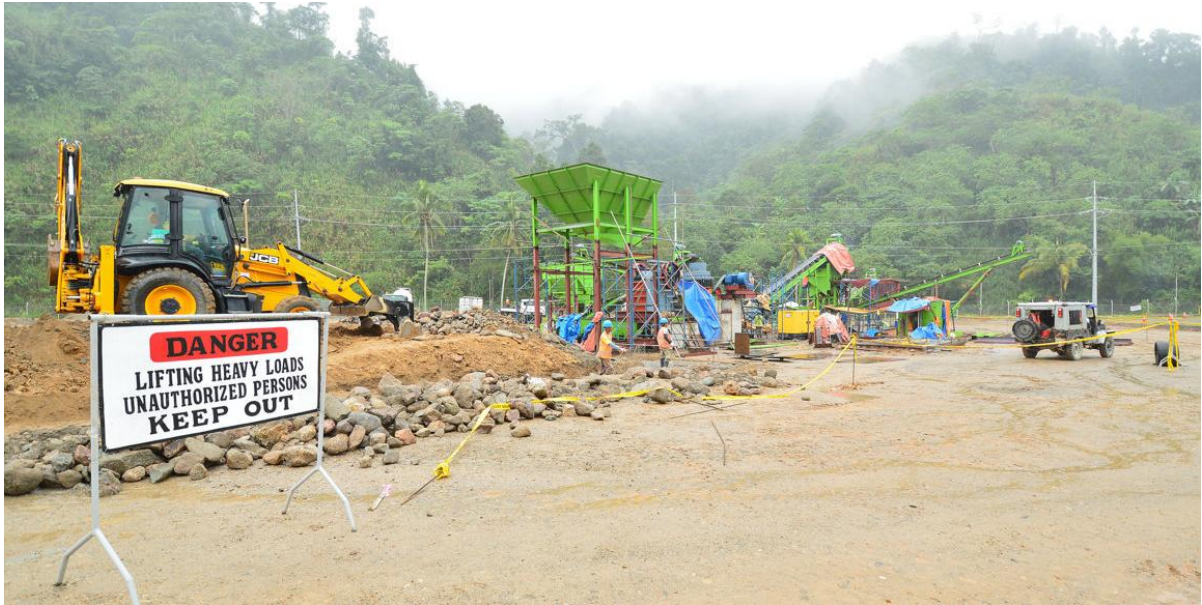
Image6. Aggregate crusher construction
