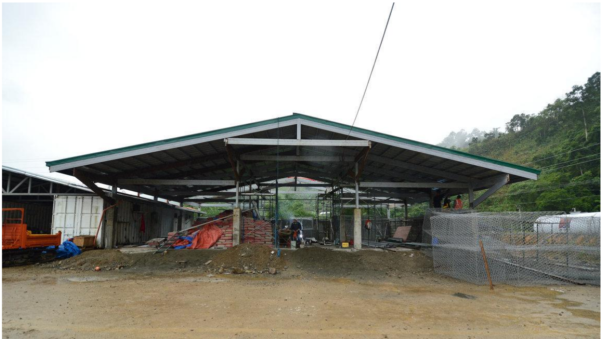
Image 4. Store and warehouse – in construction
