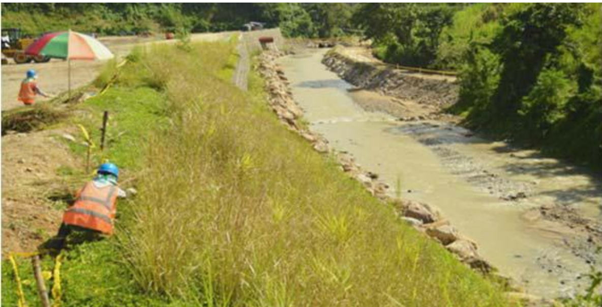
Image 14: Rehabilitation works in progress
