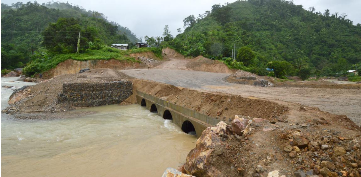
Image 10: Causeway across the Sulong River looking into Residual Storage Impoundment site – river in high flow
