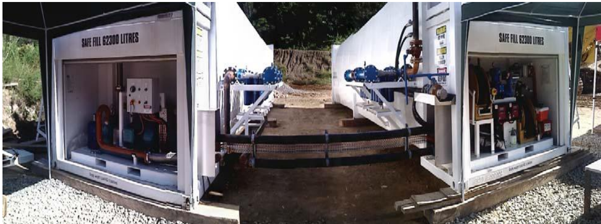
Image 8. Two diesel fuel storage tanks in situ, each with a holding capacity of 62,300 litres
