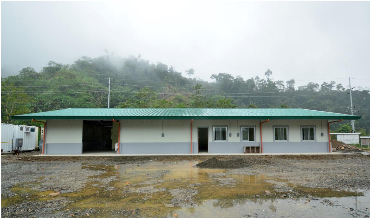
Image 3. Laundry and Camp Office Complex
