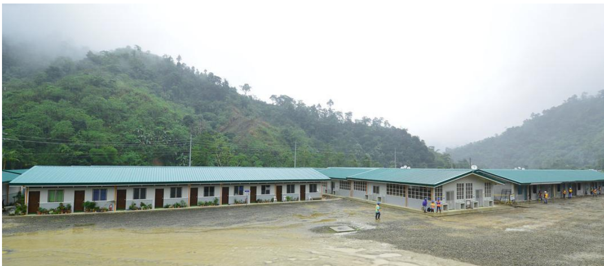
Image 2. Construction camp – ablutions (far left), accommodation and messing facilities (central building)
