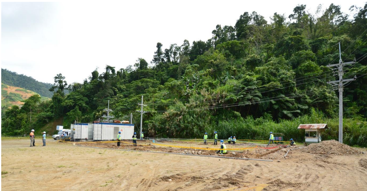
Image5. Back- up power, 2kVA installed, preparations for a further 4 kVA in progress
