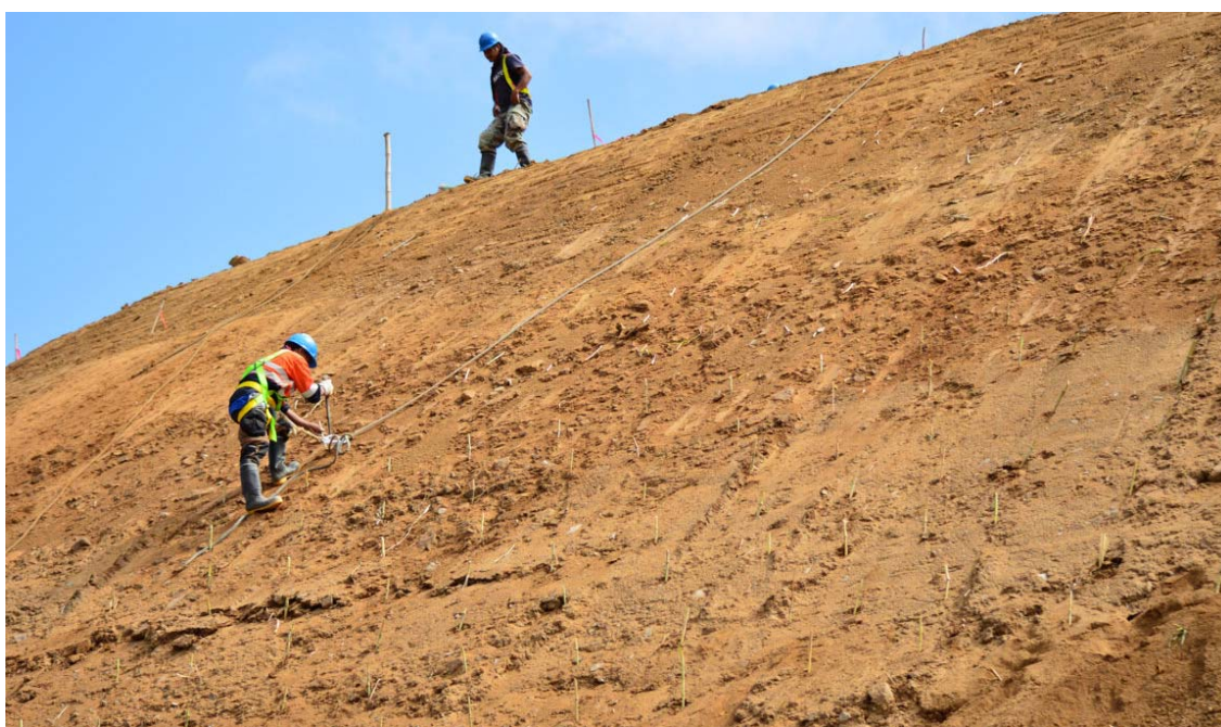
Image 12: Rehabilitation and stabilisation of a stacked surface
