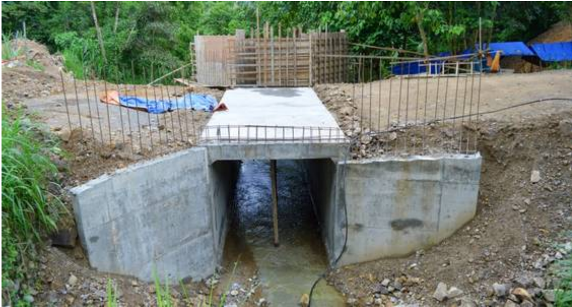
Image 9. Box Culvert, Solano – Runruno Road
