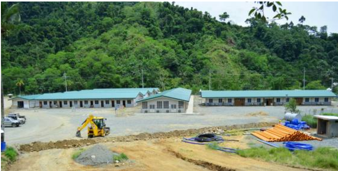
Image 4. Construction camp - ablutions, accommodation and messing facilities (central building)
