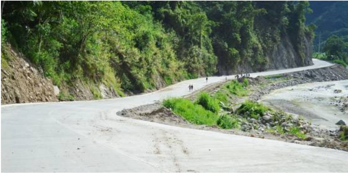
Image 10. Road Rehabilitation_Solano – Runruno Road – Concrete Surfacing by DWPH, Solano
