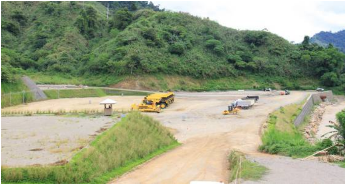
Image 2. Processing plant pad viewed from the mine "starter pit" area
