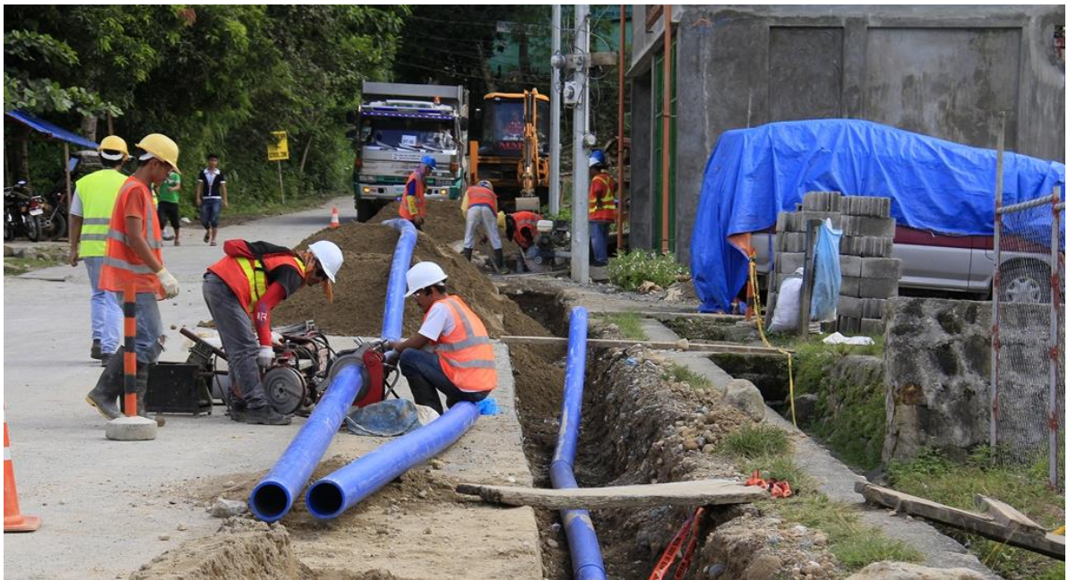
Image 9. Laying potable water pipe line through Runruno township
