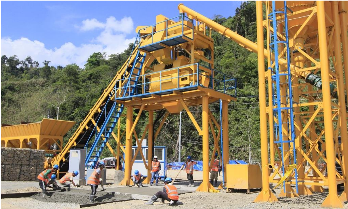
Image 10. Concrete Batching Plant
