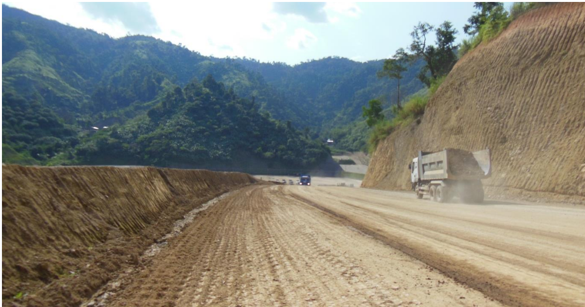
Image 12. Mine haul road
