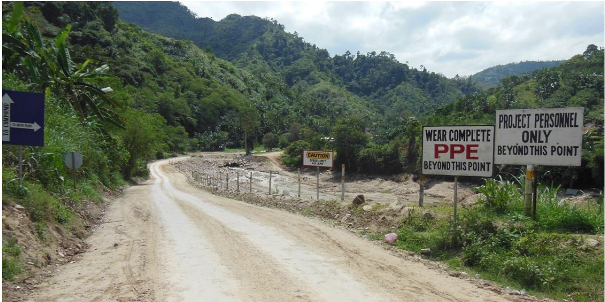
Image 1. Site access road - looking towards campsite and lay-down area
