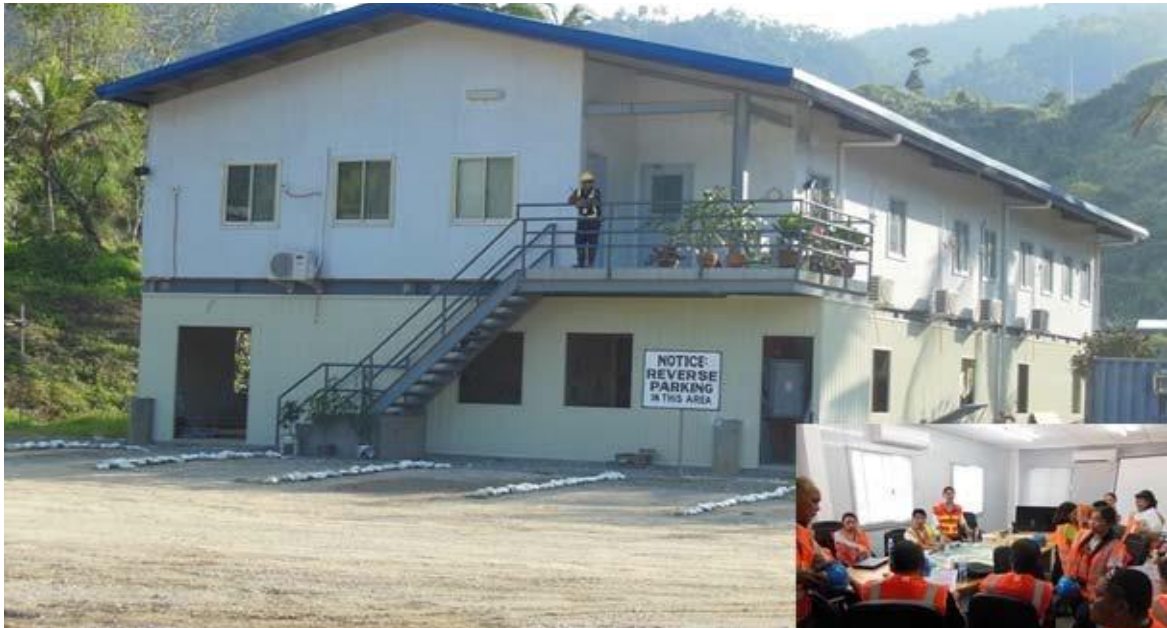
Image 3. Two storey office block
