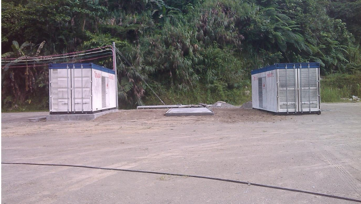
Image 7. Construction generating capacity – Two 1,000 kVA units
