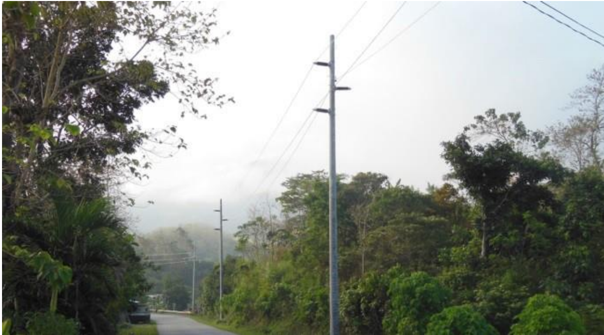
Image 8. Stage One – 69kV power line Runruno to Maddiangat
