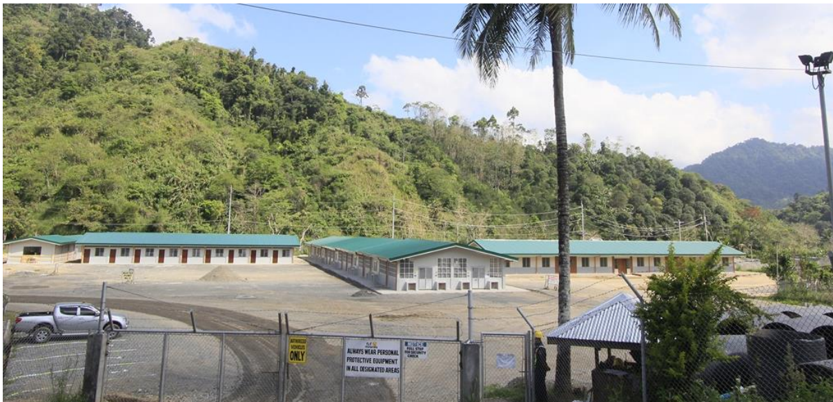
Image 4. Construction camp - ablutions, accommodation and messing facilities (central building)
