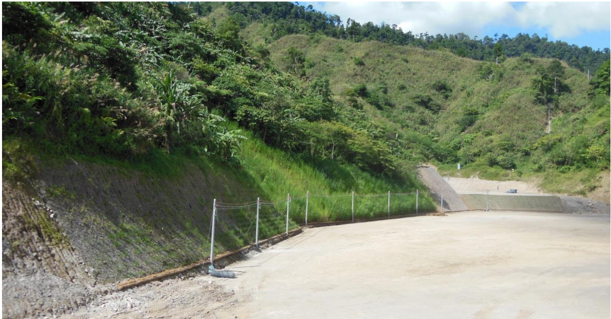
Image 6. Construction power reticulation
