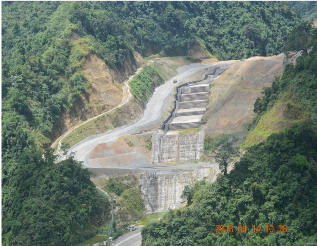
Residual Storage Impoundment – spillway view
