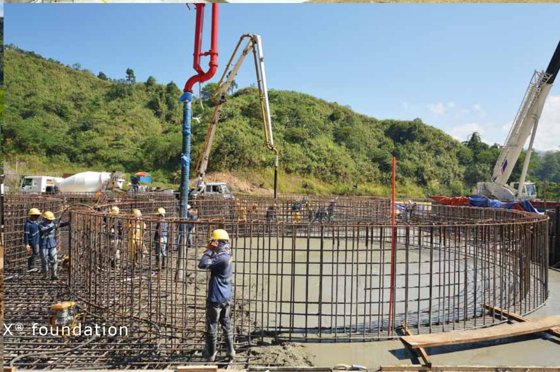
Construction of Counter-Current Decantation (CCD) Thickener foundations
