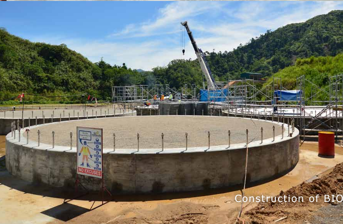
Construction of Carbon-in-Leach foundations
