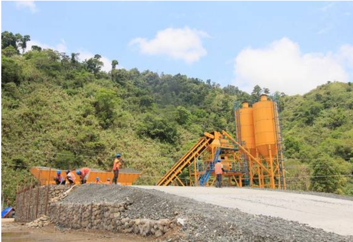
Picture12 – assembled batch plant on site ready to produce and pour concrete
