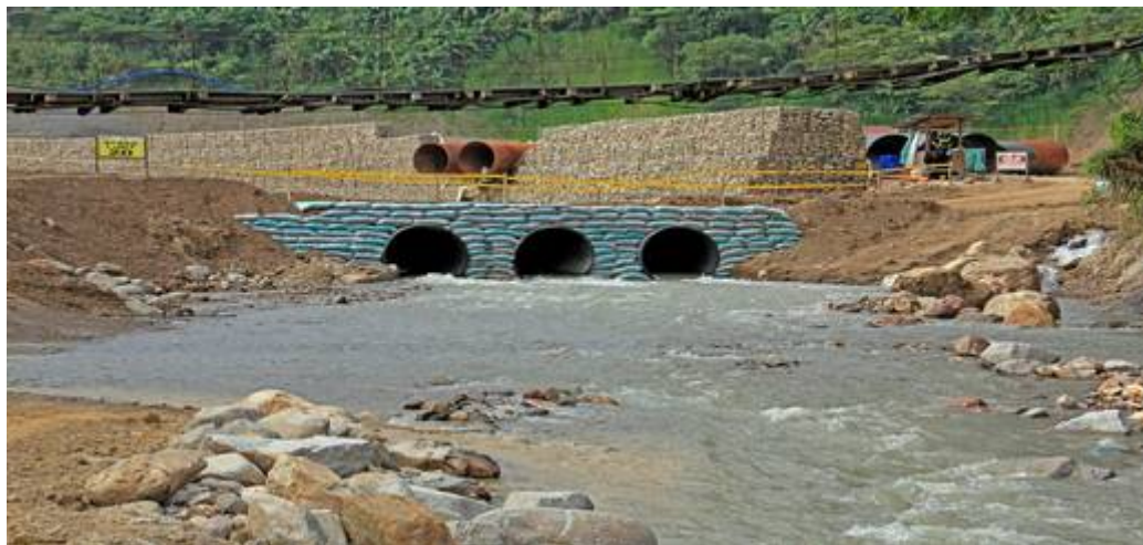
Picture4– gabion baskets strengthening the Sulong river bank
