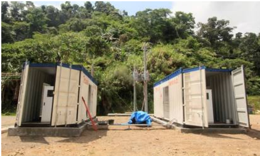
Picture10 – backup and standby generators in-situ
