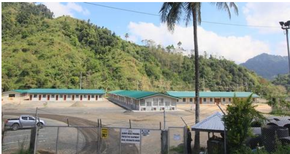
Picture8 - Construction camp - ablutions, accommodation and messing facilities (central building)
