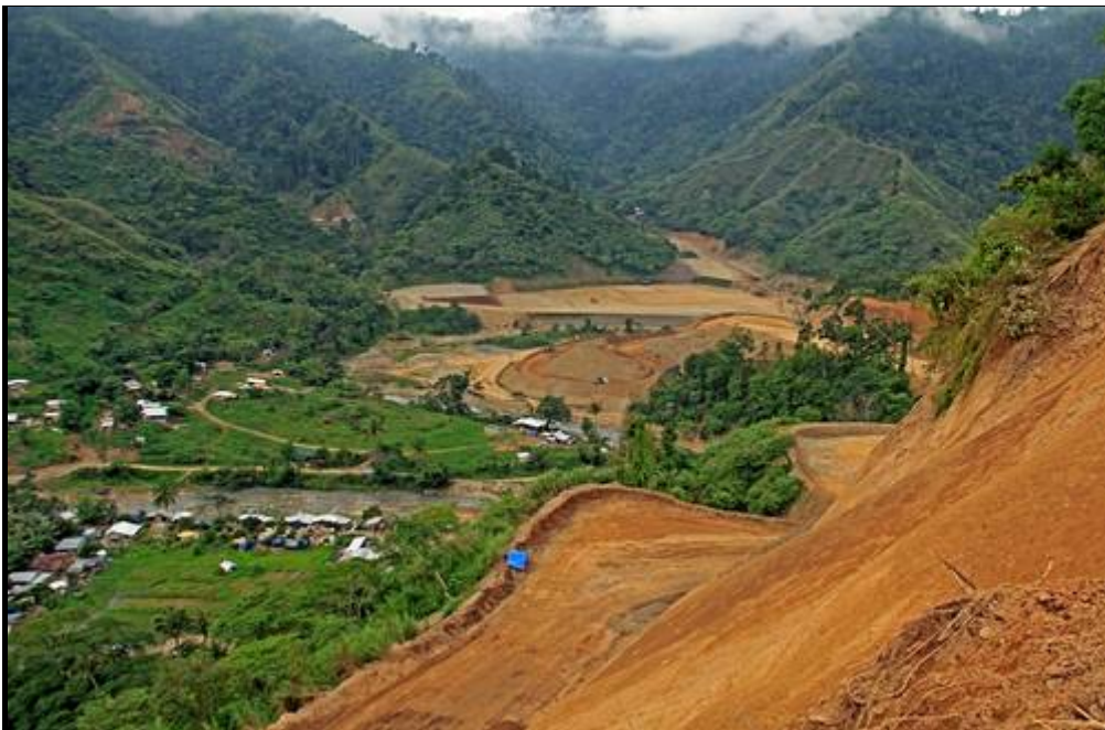
Picture14 – haul road aerial view
