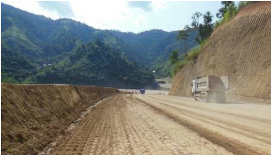
Picture16 – haul road April 2013
