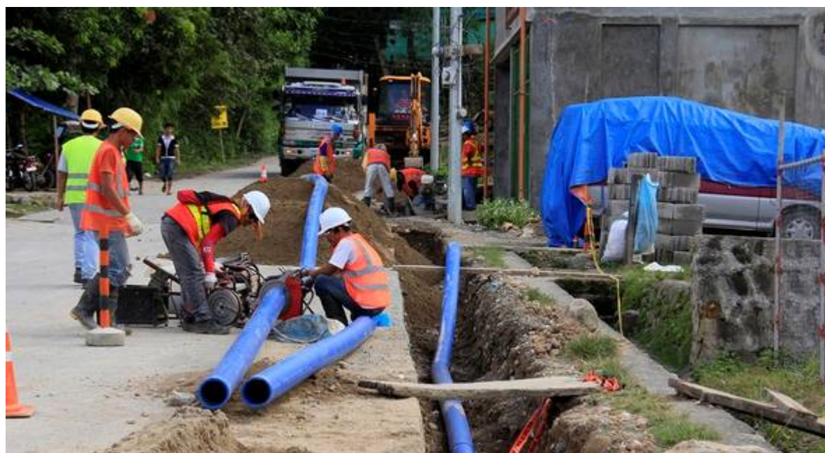
Picture11 – laying the water mains pipe
