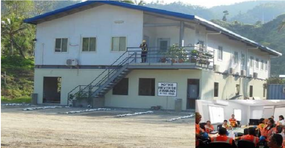
Picture7 – two storey office block
