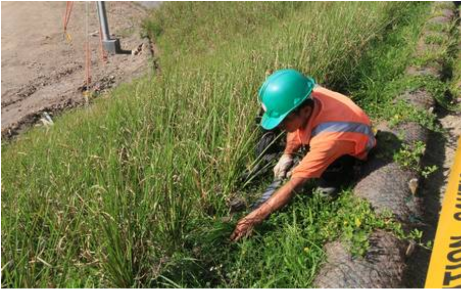
Picture5 – rehabilitation & strengthening earth slopes around the processing plant site
