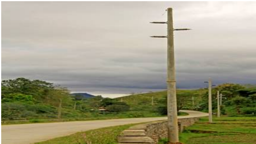
Picture9 – new electricity poles in-situ
