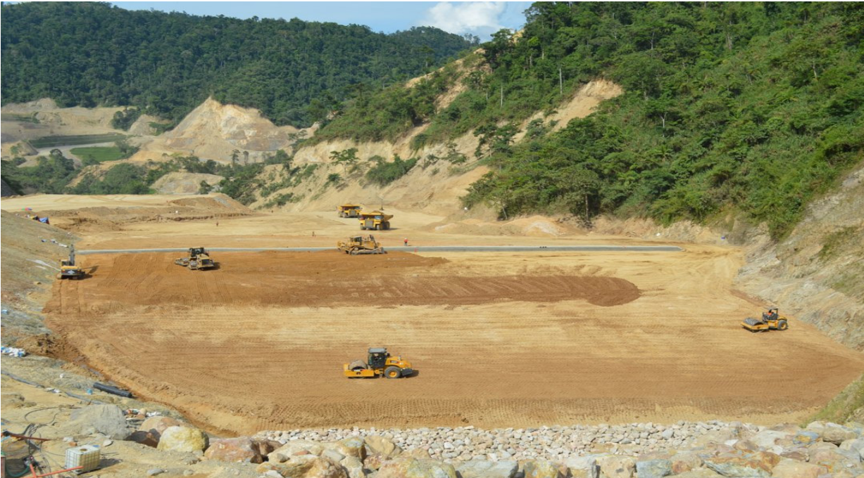
Construction works in the Residual Storage Impoundment – May 2015
