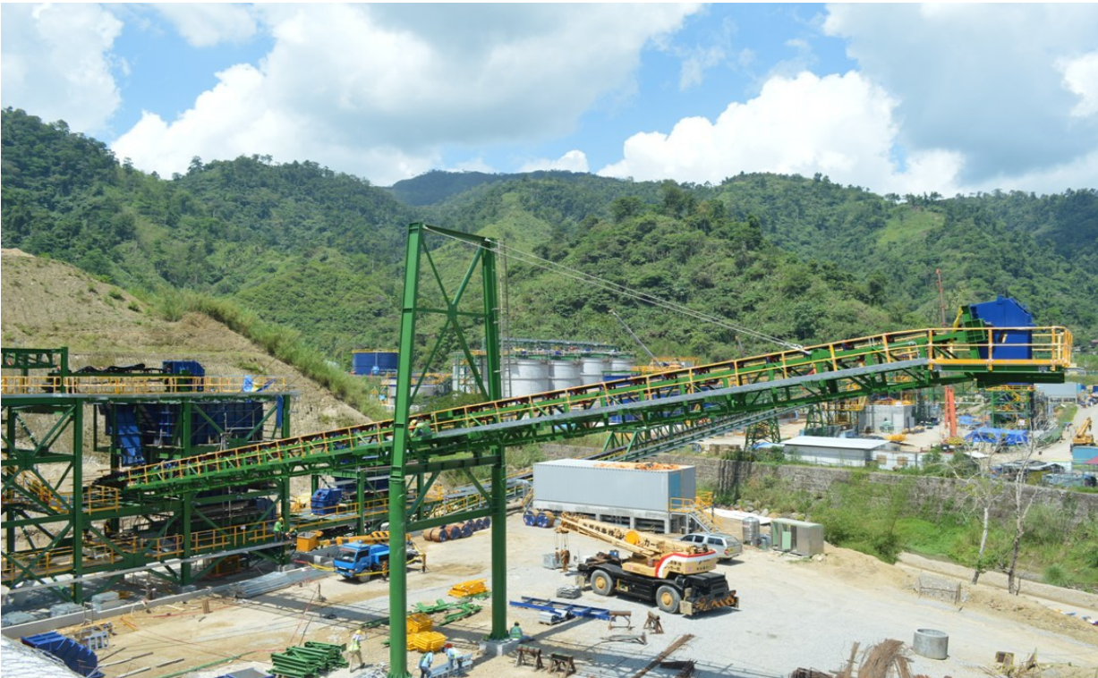
Stockpile conveyor – May 2015
