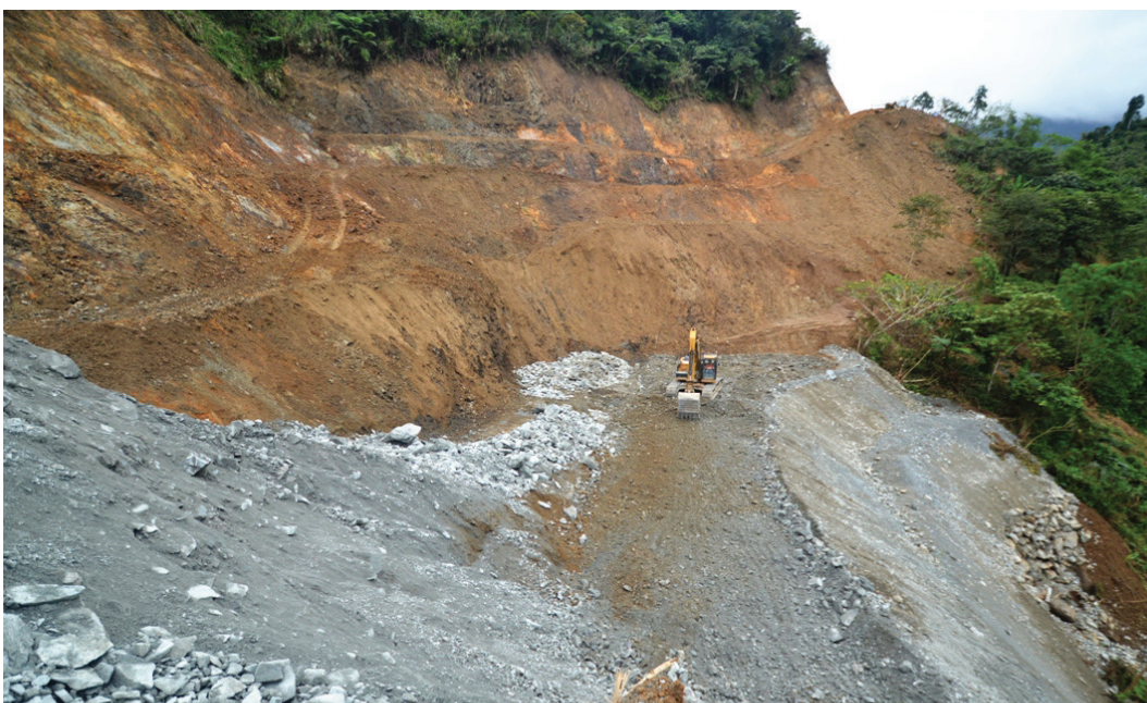
Preparation works on the Tullangan Dump Site access road, December 2017.
