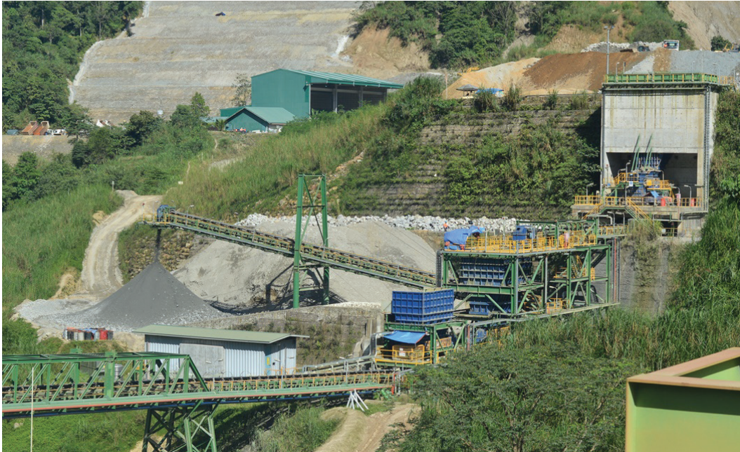
The Primary Crusher, April 2018.
