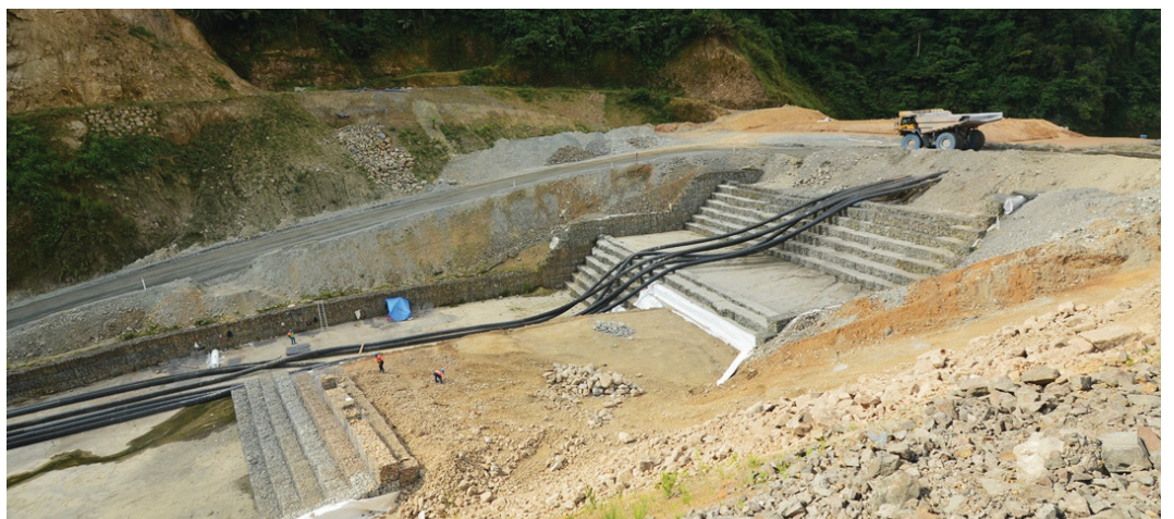
RSI spillway April 2018.
