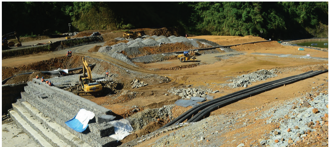
RSI spillway being constructed May 2017.
