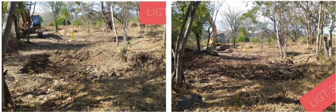
Photograph 3.1.1. (c) Remediation of mud pit in platform LIGT391
