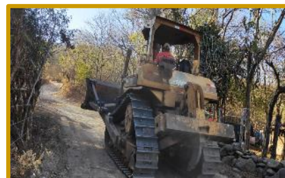
Figure 41: D6 tractor already working on road improvement
