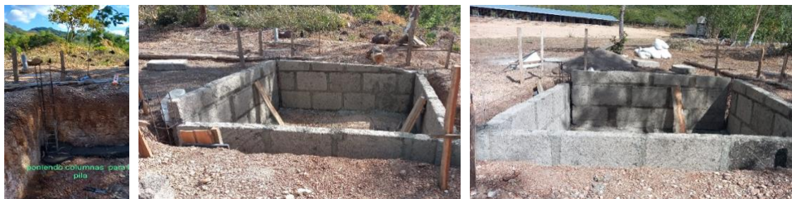
Image 3.2.5 a. Progress in construction of pit for organic waste management - compost.
