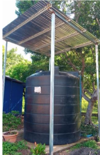
Construction of a booth in a treated water tank.
