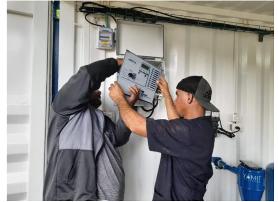
Preventive maintenance to the water treatment plant.
