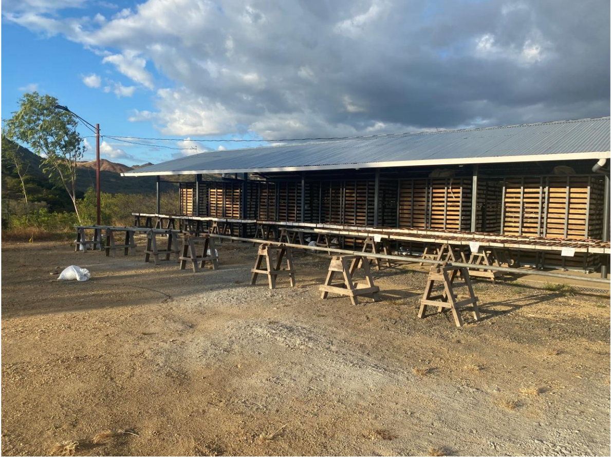
Figure 10-5: Core Laydown Facility at the La India Project Site (June 2022)
