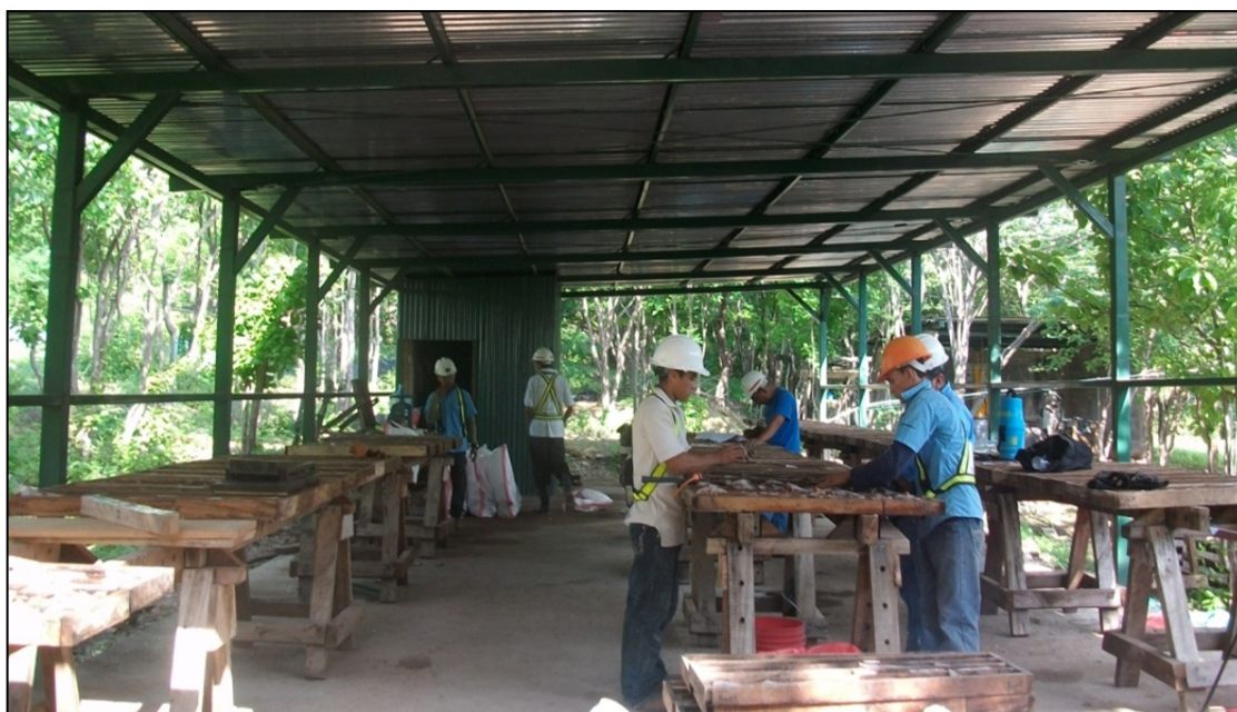
Figure 9-5: Core Laydown Facility at the La India Project Site (June 2012)
