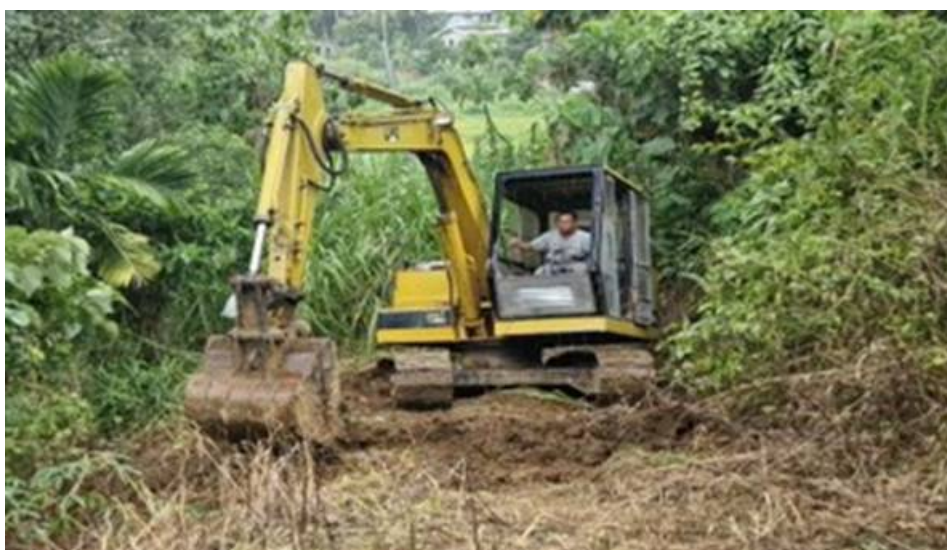
Figure 5: Access track and drill pad construction has commenced at Dupax.
