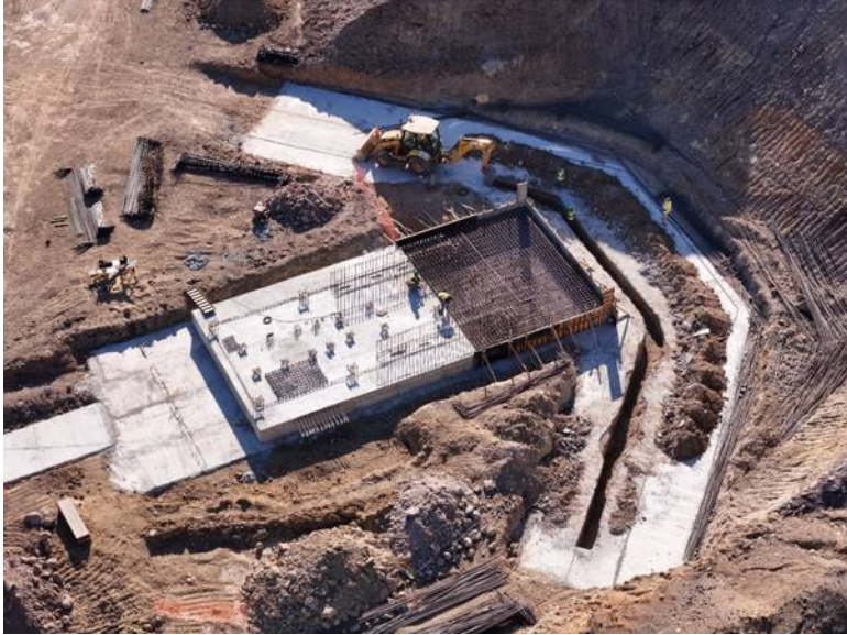
Figure 4: ROM crusher footings and wing wall
