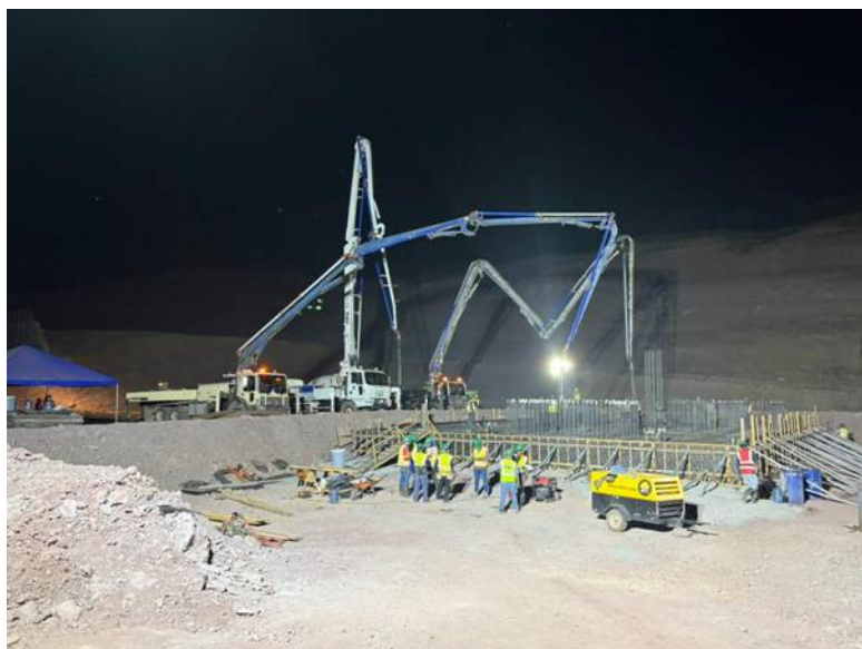
Figure 2: Concrete pour mill footing and raft beam
