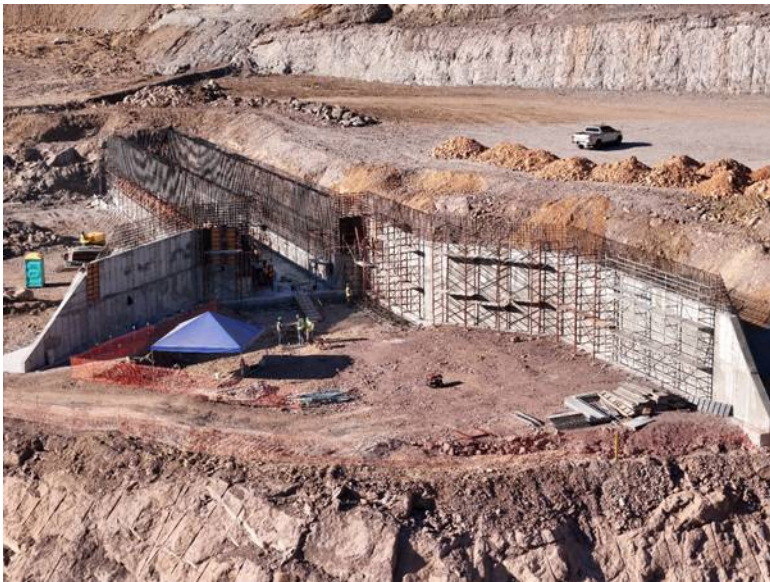
Figure 5: Concrete works at the Reclaim tunnel
