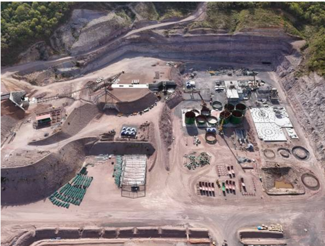
Figure 1: Overall Plant View
