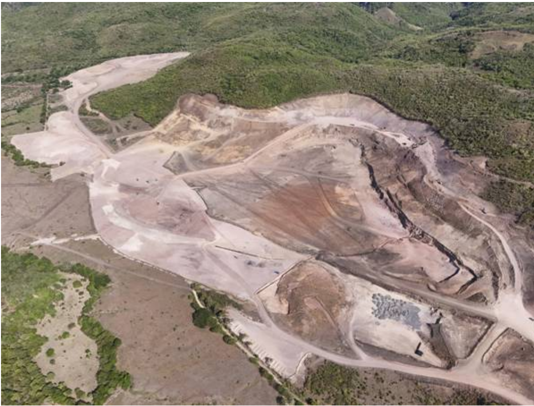
Figure 4: Tailings Storage Facility
