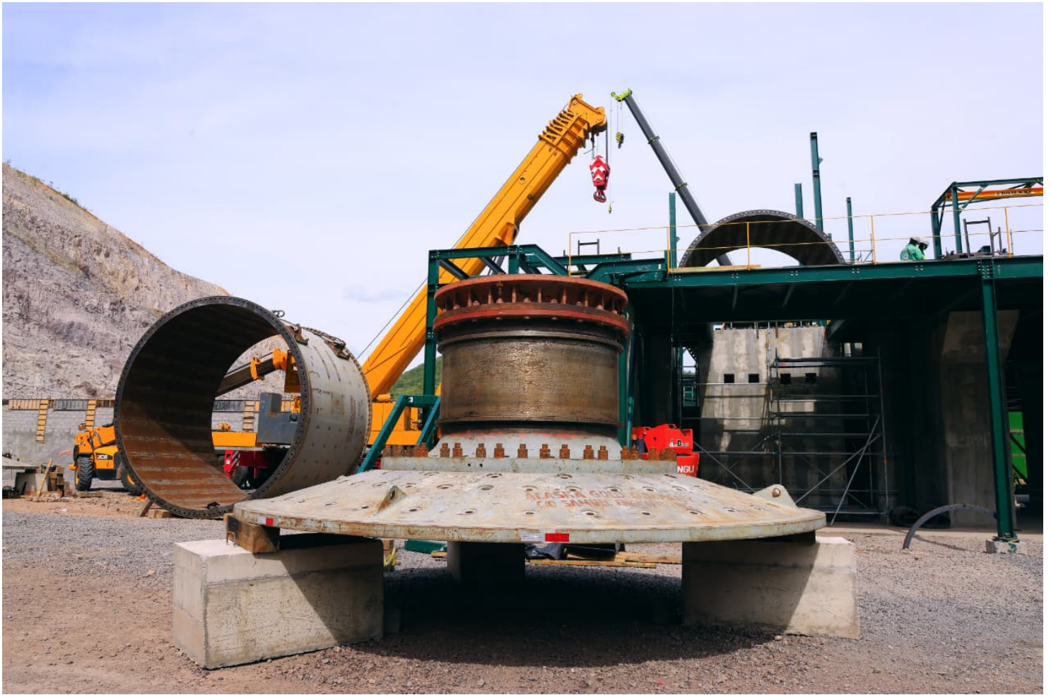
Figure 4: Ball Mill Head
