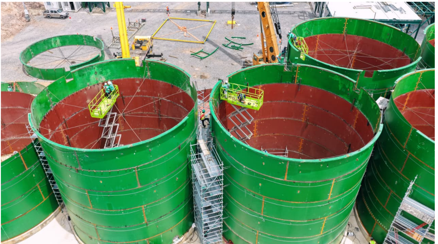
Figure 7: CIL Tank Installation
