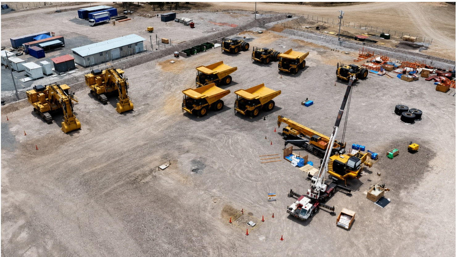
Figure 13: CAT Mining Fleet Assembly & Commissioning
