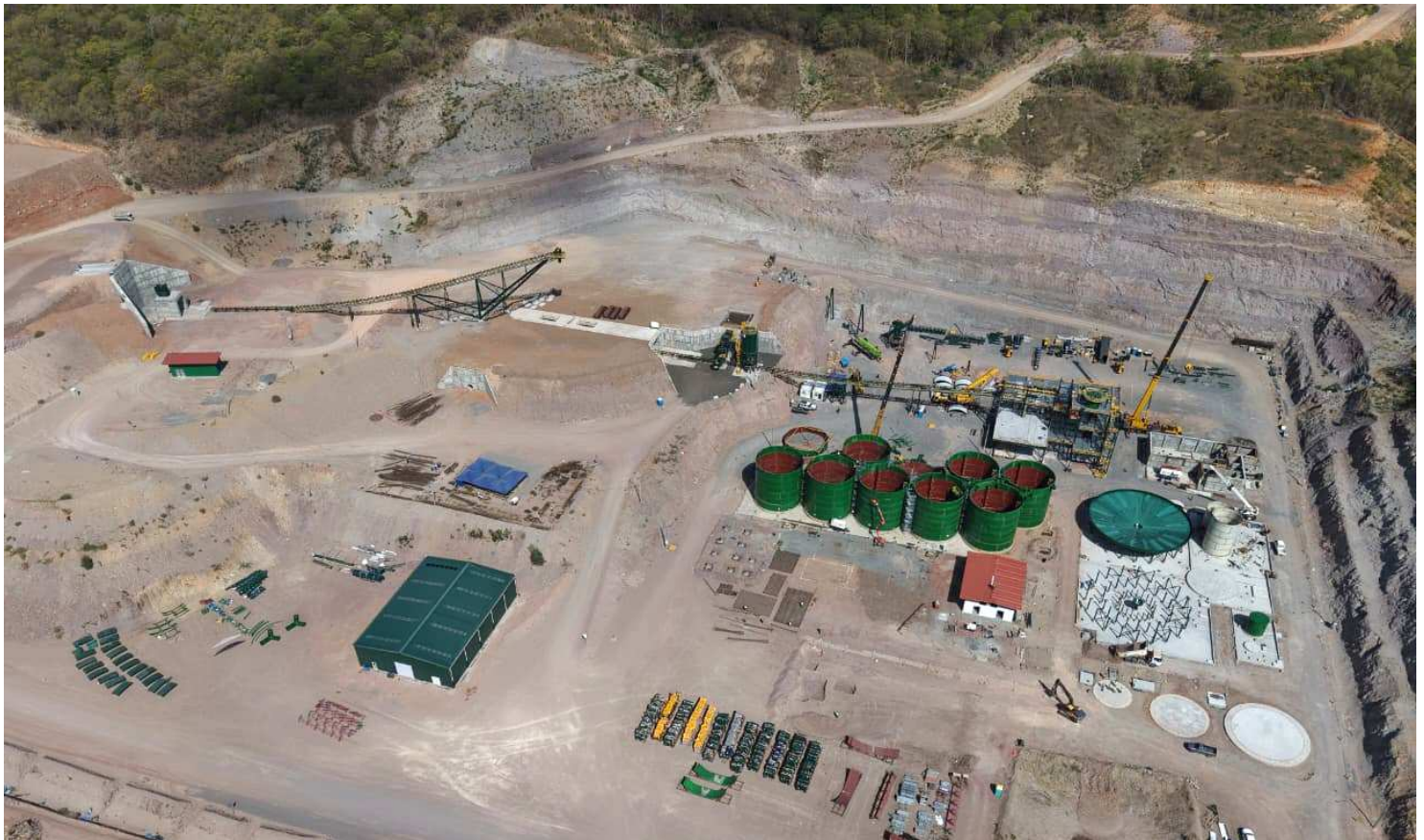
Figure 1: Overall Plant View
