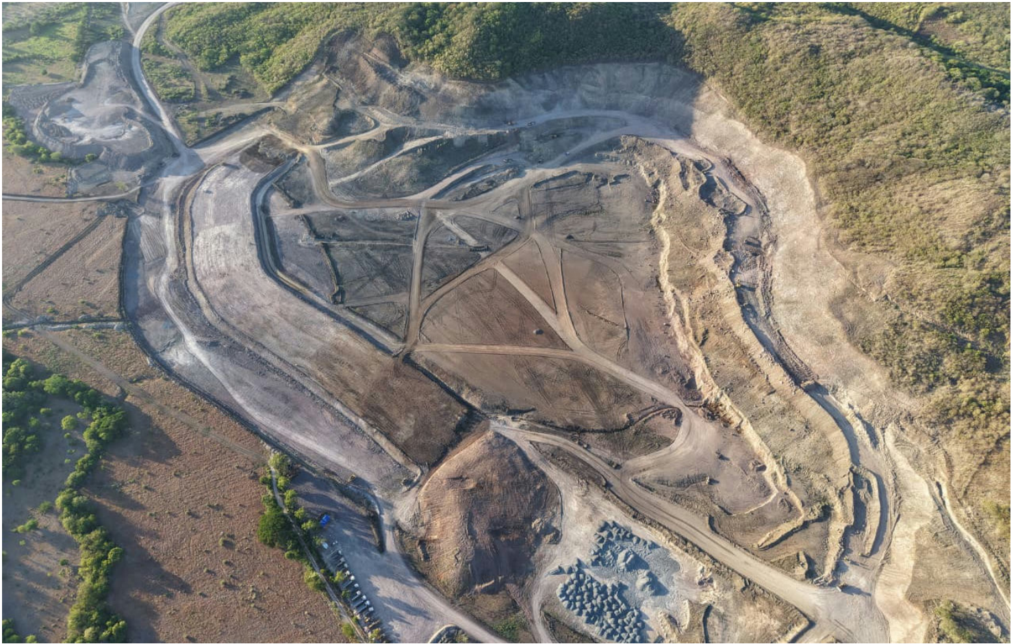
Figure 12: Tailings Storage Facility
