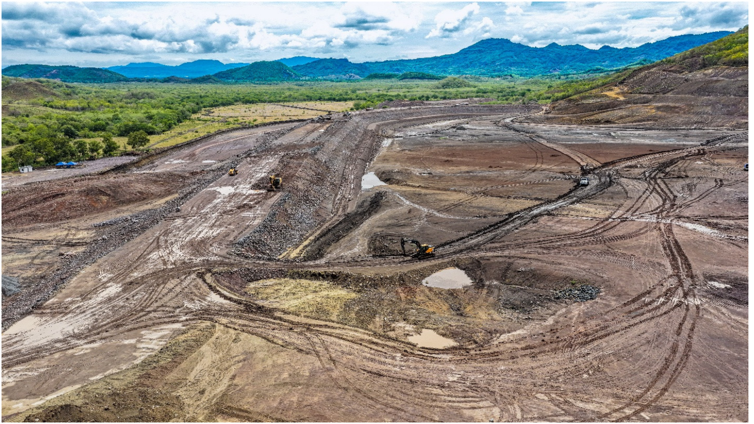
Figure 5: Tailings Storage Facility
